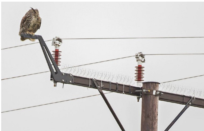
Fig. 8. Eagle-Owl perching on a power-pole with deterrent devices fitted. Photo: Karl-Otto Jacobsen.
